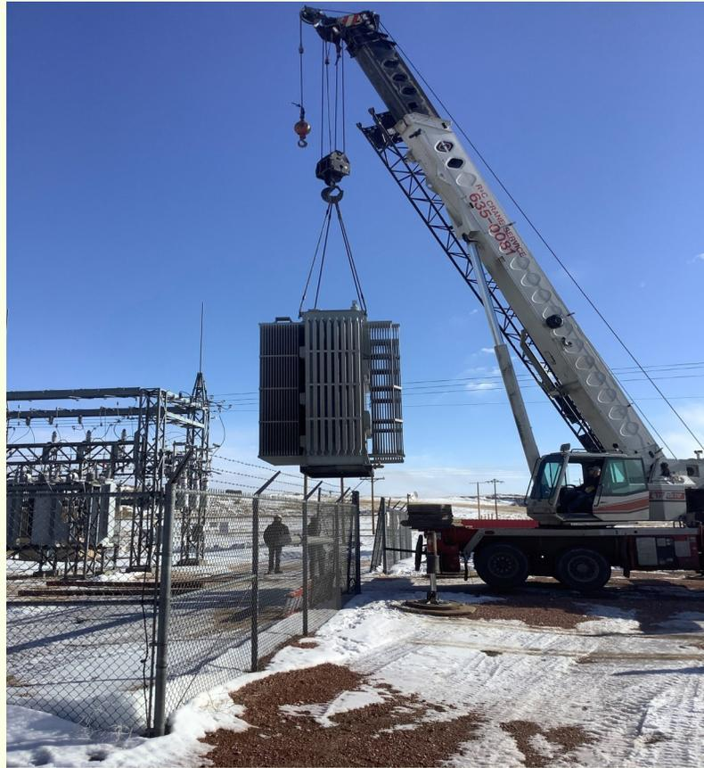
Craning of the replacement substation transformer.
