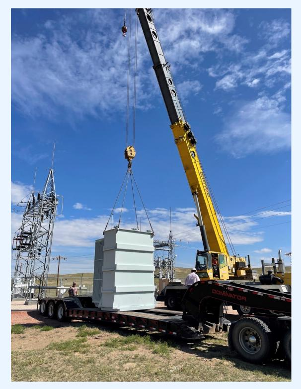
In above photo, the setting of a 5 MVA substation transformer, weighing approximately 23,000 lbs on a trailer owned by Miller Enterprises. This transformer will have to be untanked before an evaluation can be conducted at T&R Electric; a process that will take approximately 6 months. R and C crane did the lift of the transformer. Justen Miller hauled the transformer to T&R Electric in Coleman, SD to be evaluated. We are hoping simple repairs can be made.
