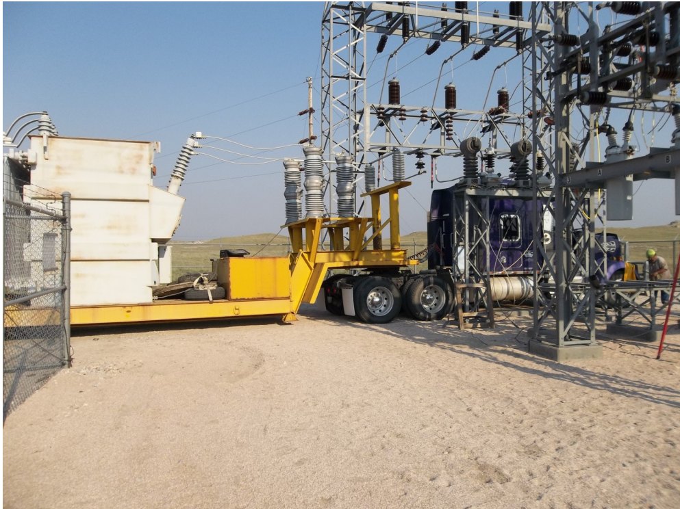
On June 28, 2012, a portable sub was trucked in to the Van Tassell Substation.
