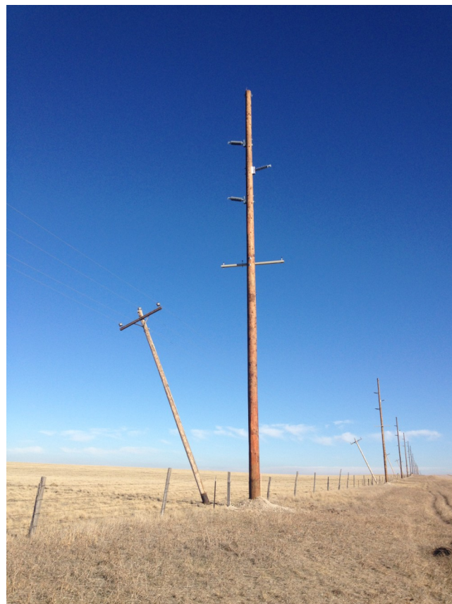
Pictured above: New 75 foot poles on Kirtley road, replacing the old 35 foot poles.
