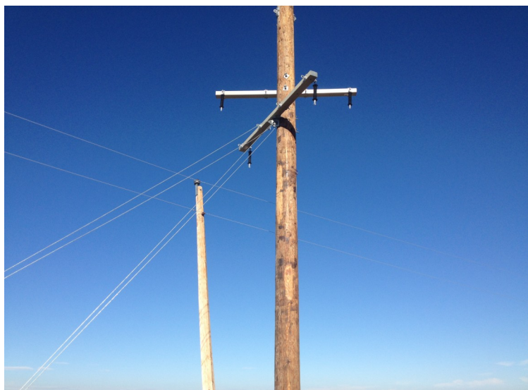
Pictured above: New 75 foot poles on Kirtley road, replacing the old 35 foot poles.
