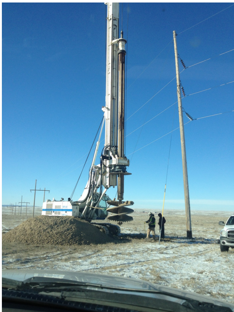
Pictured left: A 6 foot diameter auger drilling a 22 foot deep hole for steel transmission line poles feeding the ONEOK substation.
