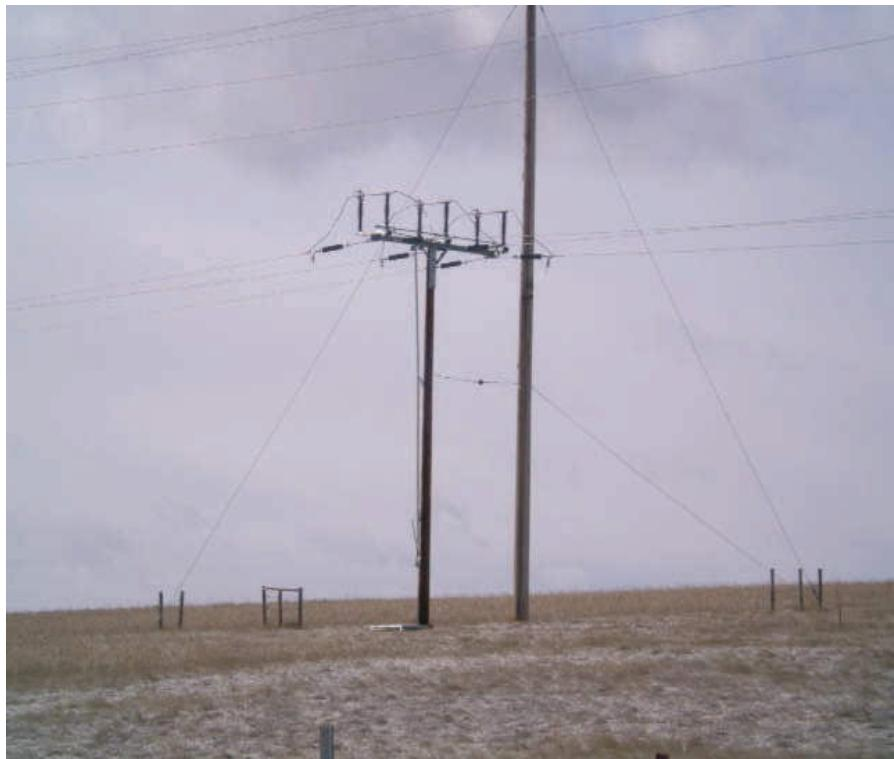
In January, NEA's 69 KV line switch installation was completed, just south of Meridian RD, off of HWY 85. The new switching gear (pictured above) allows NEA to open the line going to the Cheyenne River pump station without having to take an outage by killing the Lance Creek and Hat creek substations.
