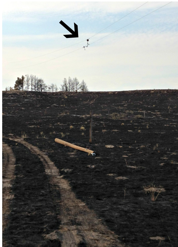
Below Right: The arrow points at some pole hardware still clinging to the line. A new pole lays on the ground waiting to replace the burned stump next to it.
