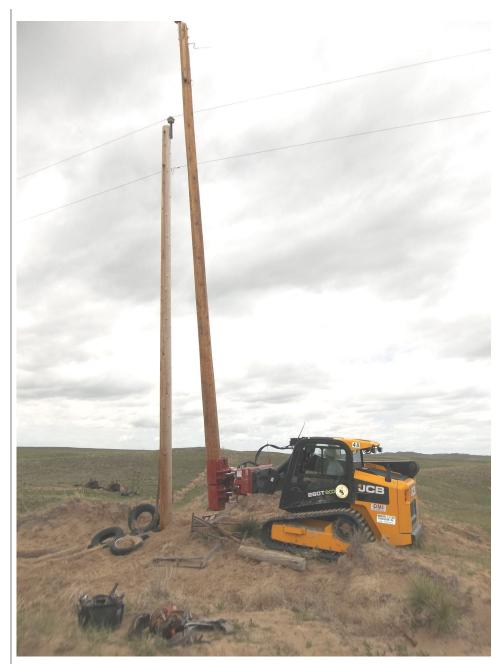
Line crews have been busy putting the versatile, new equipment purchased by NEA to use. As seen above, the detachable pole grappling device works beautifully to set or remove poles. On page two, Nebraska Linemen Matt Edwards and Justin Huston use the detachable auger unit for drilling pole holes.
