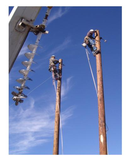
This year, pole testing was done in the Lusk to Node area and south. Approximately 100 of the 3900 poles inspected/tested, failed, or about 2.5%. Add to that some that tested "soft", shell rotted or other issues noted, and we will be replacing 150-200 poles next year. We fell behind with the blizzard of 2013, so we were replacing 2013 and part of 2014 failures this spring and hope to get caught up on the rest of the 2014 poles with this group.
