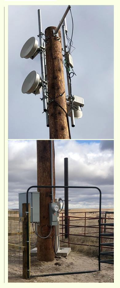
Photos Left: A collector box, which holds meter readings, hangs on the side of this pole and from the meter running up the pole is an antenna that rises a few feet above the 65ft pole. At the top, sharing space on the pole, Vistabeam's equipment supplying internet to the area and sending our meter signals to a Landis & Gyr service center in Kansas.
